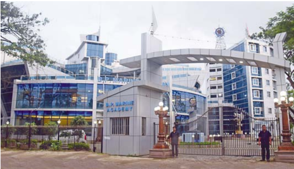
B. P. Marine Academy, Phase – I Panvel Campus Facility
